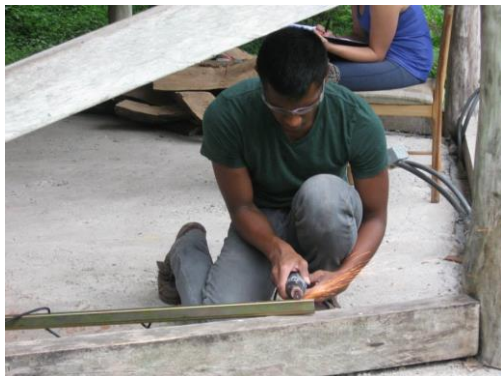
PET Thatch Roof Design Lead Deepak Ravi helping with construction.
