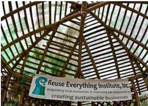
The roof built by Carnegie Mellon students in Ecuador.
